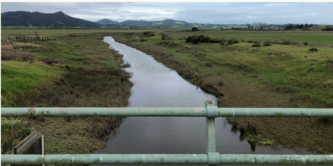
Figure 4: View of the Hikurangi swamp from Rushbrook pump station.
